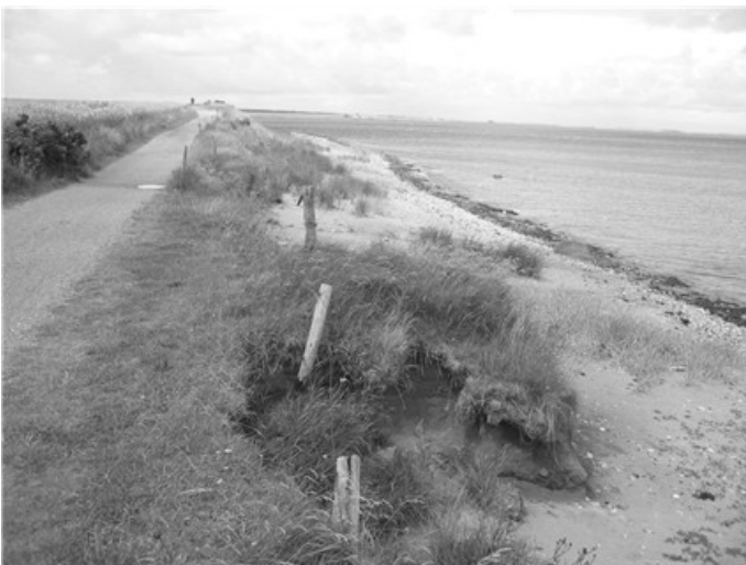
Figure 8. Erosion at the eastside of Amrum.
